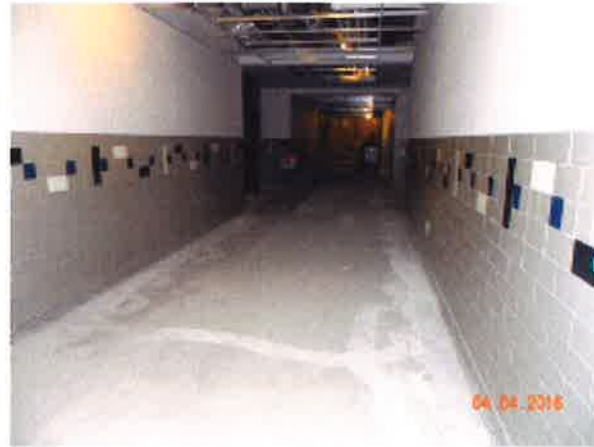
1st Floor Corridor
