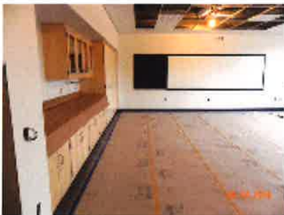
Second Floor Unit I Classroom
