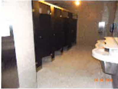
Second Floor Restroom
