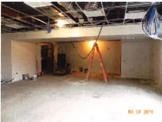
First Floor Classroom
