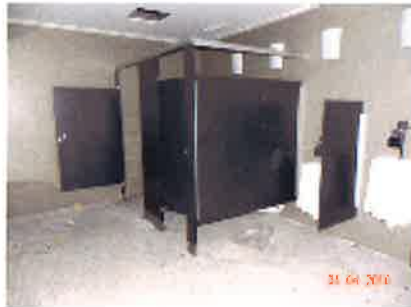
First Floor Plumbing Rough In
