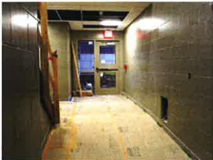
Unit I Ramp at Stairwell
