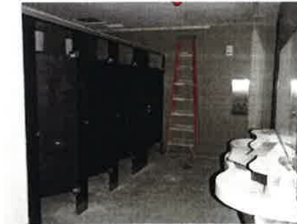
First Floor Plumbing
