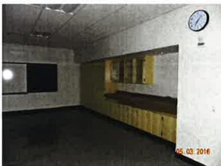
Second Floor Unit I Classroom
