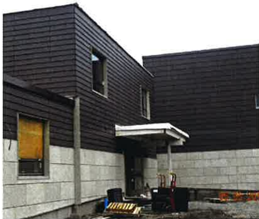
Exterior—Near Upper Gym Courtyard
