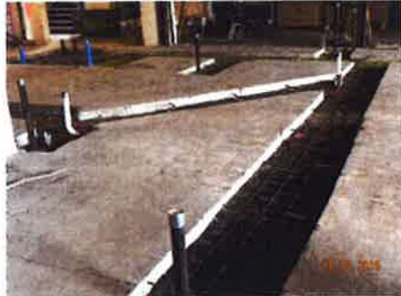
Under Slab Plumbing
