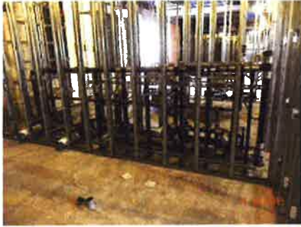
Second Floor Plumbing Rough In
