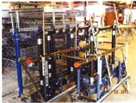
Pre-fab Plumbing For First Floor
