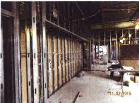
Framing Second Floor Unit I
