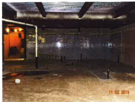
First Floor Demolition
