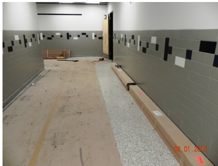
Unit C Corridor
