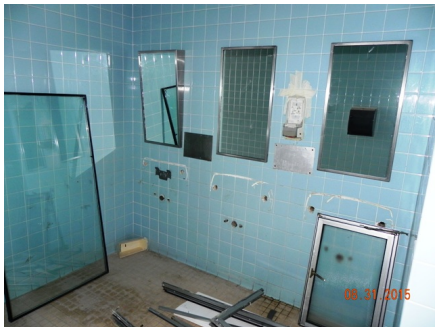
Demo 1st Floor Unit I
