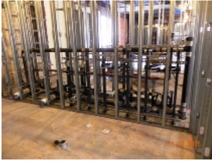
Second Floor Plumbing Rough In
