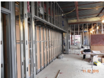
Framing Second Floor Unit I
