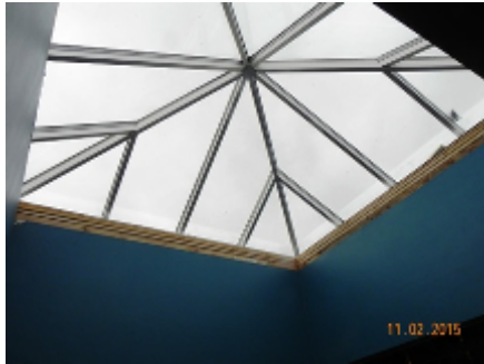
Unit I Second Floor Skylight
