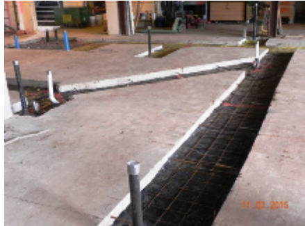
Under Slab Plumbing
