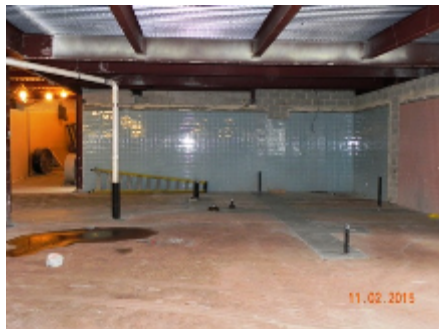
First Floor Demolition
