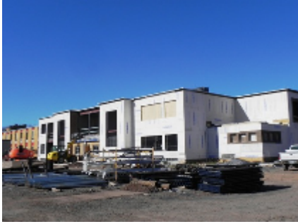
Unit I Exterior
