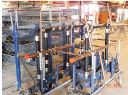
Pre-fab Plumbing For First Floor
