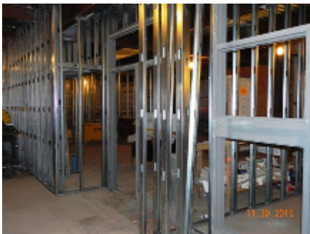
First Floor Framing
