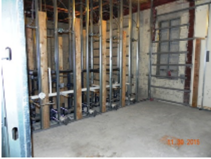
Second Floor Plumbing Rough In
