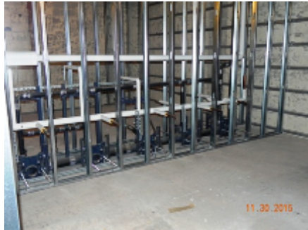
First Floor Plumbing Rough In
