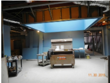
Unit I Second Floor Skylight
