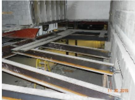
First Floor Demo for ADA Ramp
