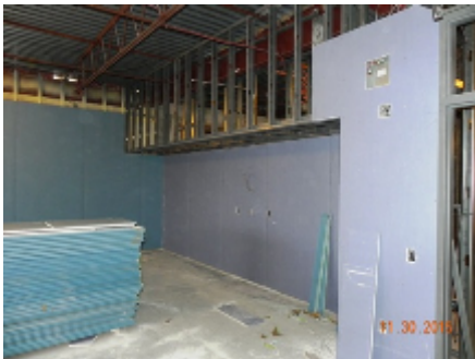
Drywall Second Floor Unit I
