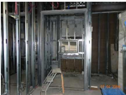
First Floor Framing Mechanical Closet
