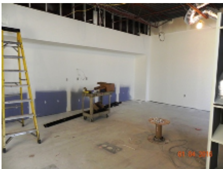
Drywall Second Floor Unit I
