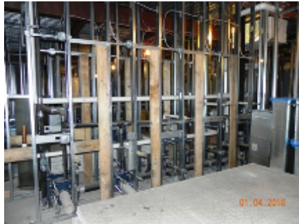
First Floor Plumbing Rough In
