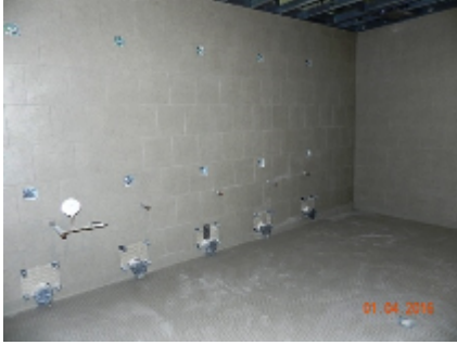
Second Floor Plumbing Rough In
