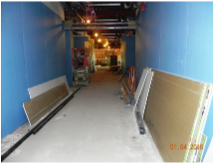
1st Floor Corridor
