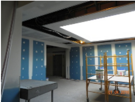
Unit I Second Floor Skylight
