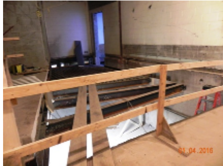
First Floor Demo for ADA Ramp
