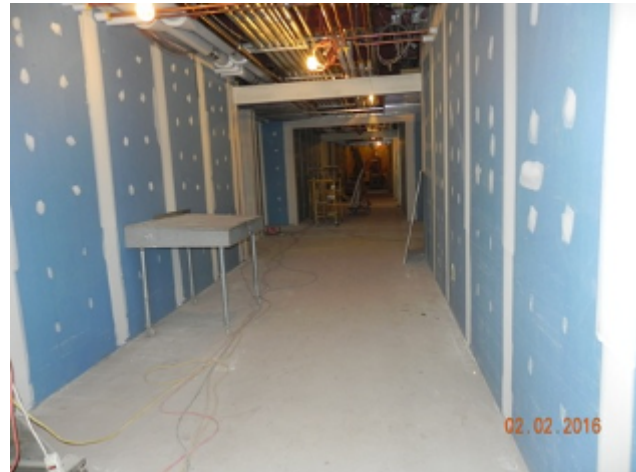
1st Floor Corridor
