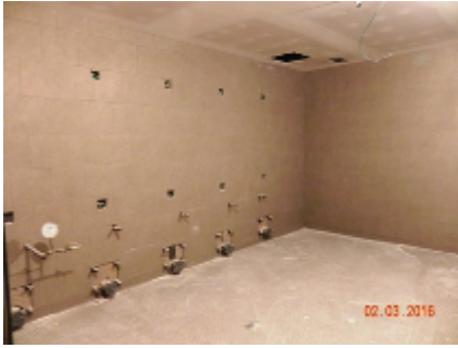
Second Floor Restroom
