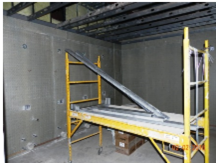
First Floor Plumbing Rough In
