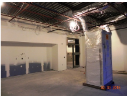
Second Floor Unit I Classroom
