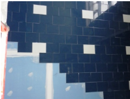
Unit I Stairwell
