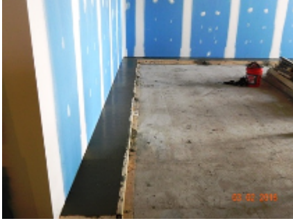
Unit I Locker Lobby
