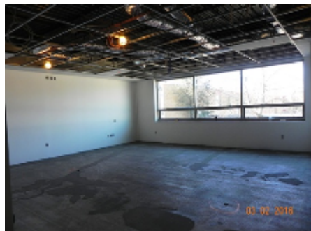
Second Floor Unit I Classroom
