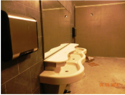
Second Floor Restroom
