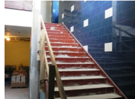
Unit I Stairwell
