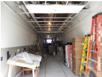
Second Floor—Unit I Corridor
