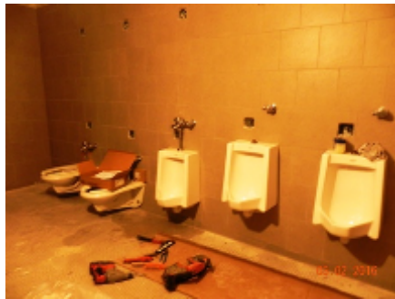
First Floor Plumbing Rough In
