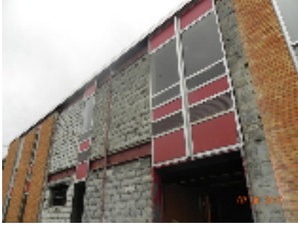
South Side Exterior Unit J (Old District Office)
